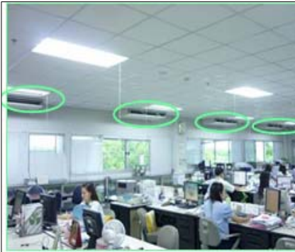
Electricity reduction 29,943 Baht/year CO2 emissions reduction 5.93 ton-CO2
