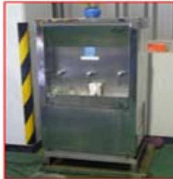
Installation a timer control at drink tank & vending machine.
