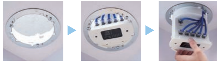
(設置・取付の様子)
