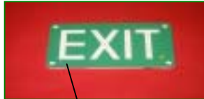
Installing of self luminous exit
